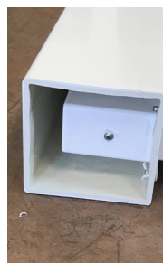
Step 7: Screw top and bottom rail into gate pockets.
