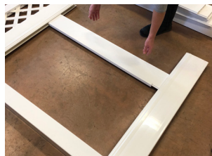
Step 4: Put U-Channel on first picket and slide into mid and bottom rail. Slide the rest of the pickets in and put other U-Channel on the last picket.
