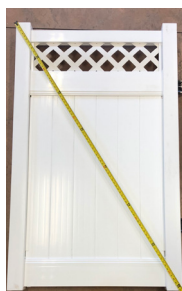
Step 6: Measure to make sure the gate is square.
