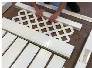
Step 1: Place lattice into top rail.
