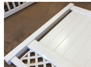
Step 5: Put top, mid-rail, and bottom rail into other post.
